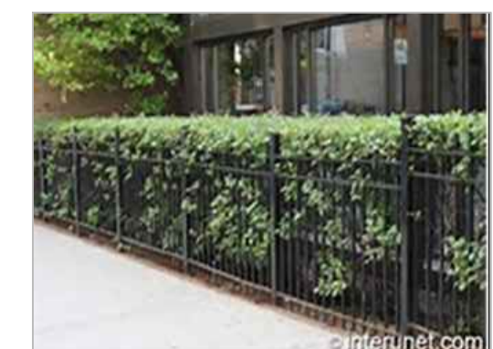
WW Rd boundary treatment Black steel railings and laurel hedge 1.2m high
